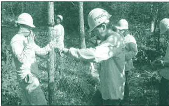
MCC crew installing deer fence
