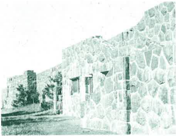
The massive retaining wall at Gooseberry Falls, known as the “Castle Wall”, was one of the largest CCC projects on the North Shore.
